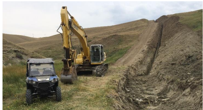
Laying of North Lateral Pipeline
