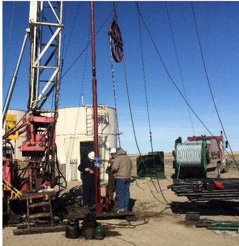
Installation of ESP in well 5991
